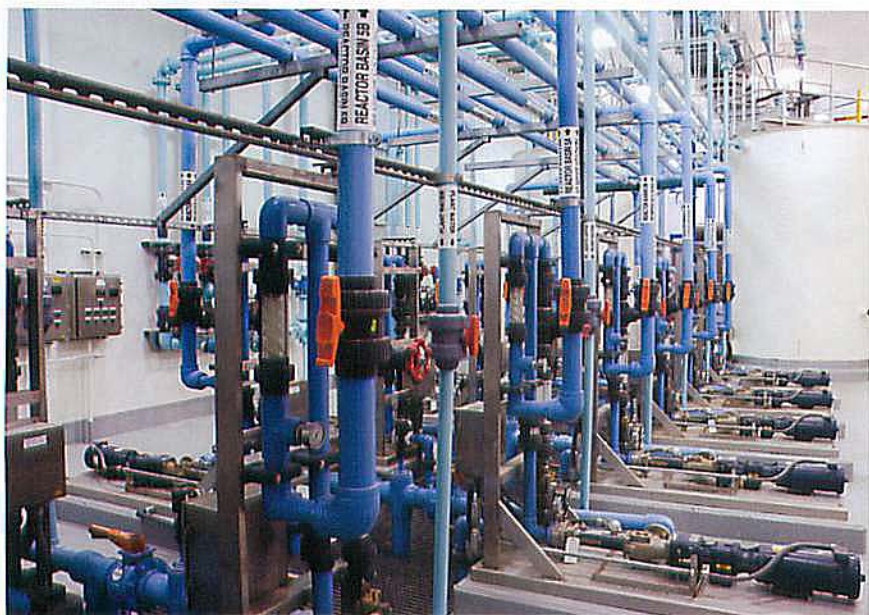
Polymer feed pumps at the CSO abatement plant.
